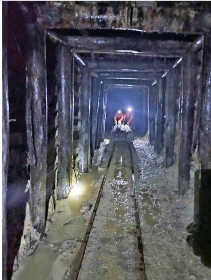
Figure 1: Photograph of underground rehabilitation work currently being done at the Bethania silver mine, Peru. Here, workers are transporting support timbers through a newly-reconditioned section of the mine.
