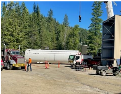
Photo 7: Lime silo being prepared for transport
