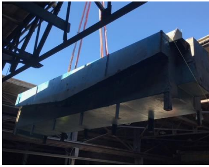
Photo 4: Flotation cell lifted through roof of Pend Oreille Mill
