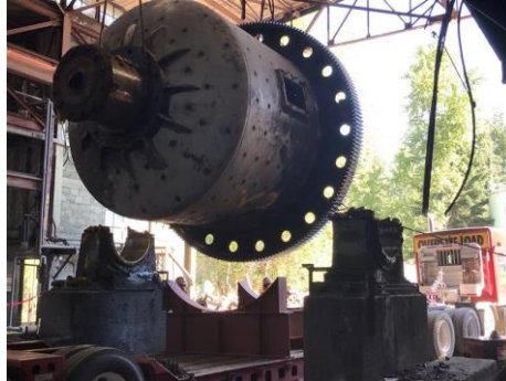
Photo 2: Ball mill hoisted by 265 ton crane
